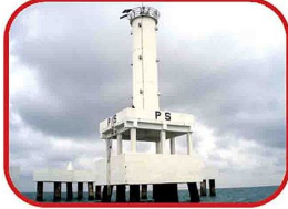
● FRP Beacon Tower (Light House) Installed At Straits Of Malacca
